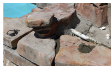
6. Extend plumbing into basin; set additional small boulders as needed.
