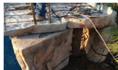
3. Bottom grotto lids rest on columns; dowel into columns.
